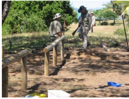
Coastal Fencing at Yarrowonga Point
