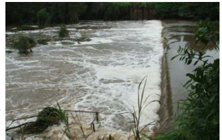
Plane Creek in flood
