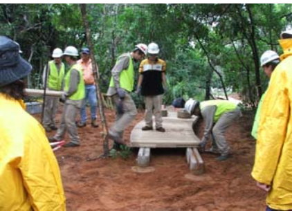
Installing boardwalk at Hay Point
